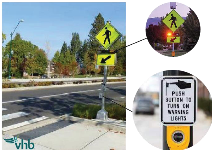
Figure 11: Example of a rectangular rapid flashing beacon.
