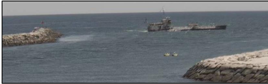
Currituck Dredging the Federal Channel
