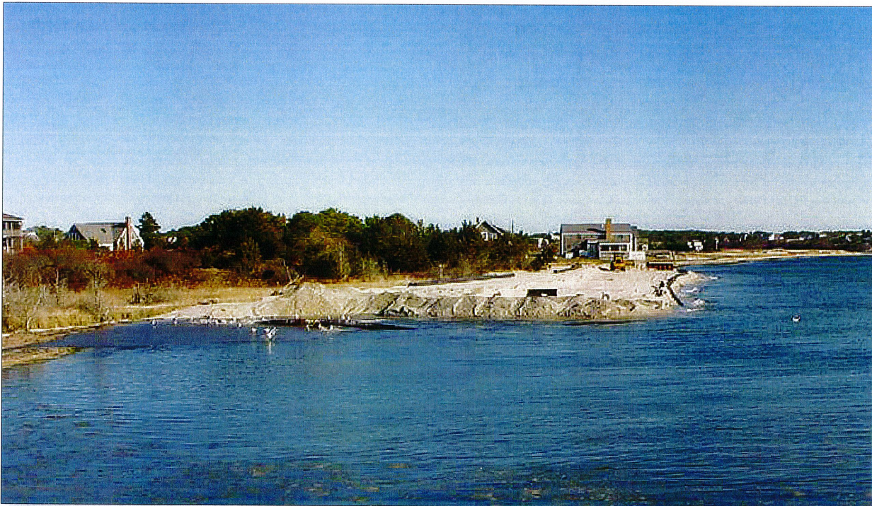
Chatham's south coast shoreline nourishment with sand dredged from Stage Harbor Channel.
