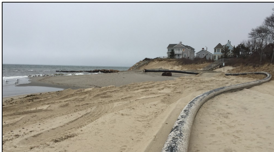
Figure 18. Lengths of HPDE discharge pipe and dewatering area, April 2017.
