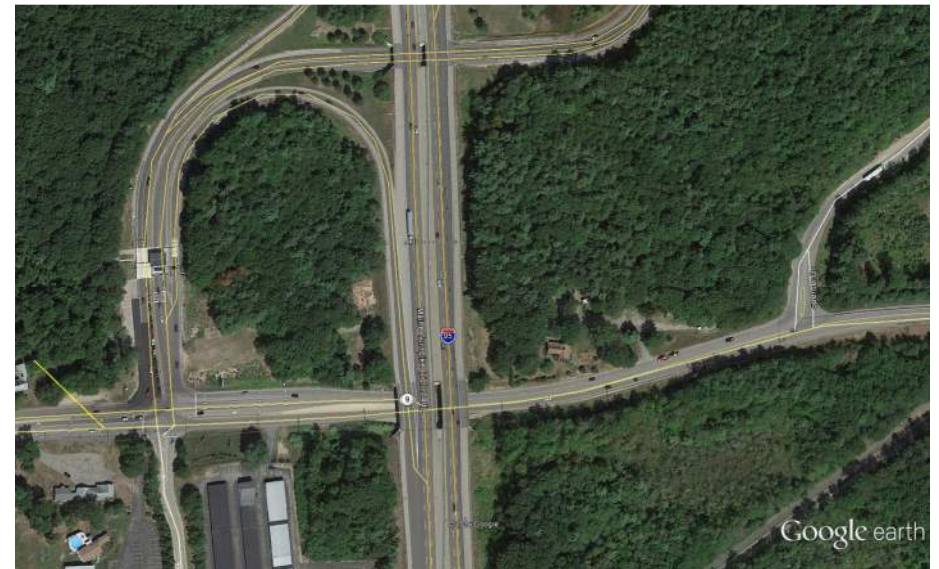
FIGURE 19: SEGMENT OF ROUTE 109 AND 9 (SANFORD ROAD) BETWEEN MTA EXIT 19/WELLS TRANSPORTATION CENTER AND SPENCER DRIVE
