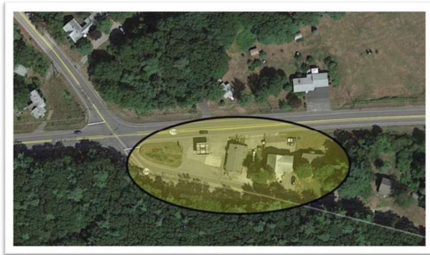
FIGURE 29: ACCESS MANAGEMENT DEFICIENCIES AT INTERSECTION OF ROUTE 109 (SANFORD ROAD) AND BRANCH ROAD/CREDIFORD ROAD
