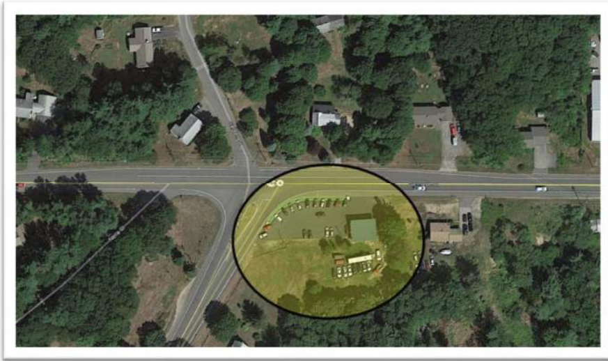
FIGURE 31: ACCESS MANAGEMENT DEFICIENCIES AT INTERSECTION OF ROUTE 109 (SANFORD ROAD) AND ROUTE 9 (NORTH BERWICK ROAD)/GARDEN STREET
