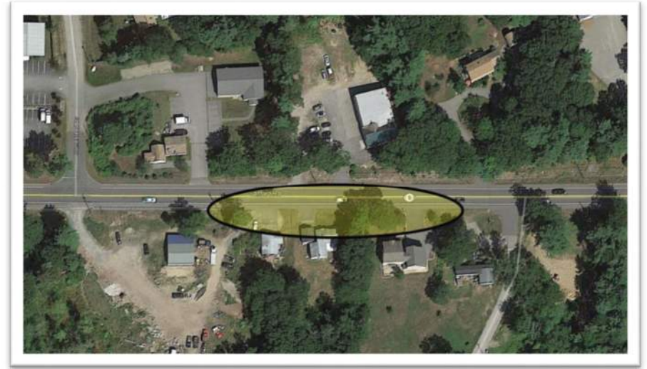
FIGURE 32: ACCESS MANAGEMENT DEFICIENCIES ALONG ROUTE 109 (SANFORD ROAD) BETWEEN INTERSECTION WITH ROUTE 9 (NORTH BERWICK ROAD)/GARDEN STREET AND MTA EXIT 19/WELLS TRANSPORTATION CENTER
