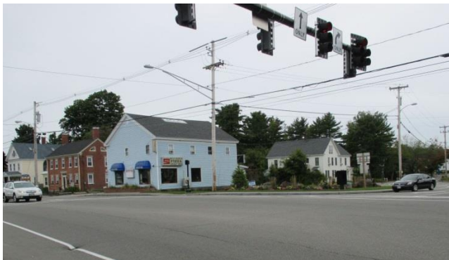
Wells Corner before Cumberland Farms construction begins September, 2014
