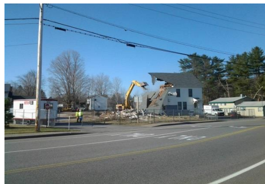
Demolition of Wells House of Pizza building on Route 109
