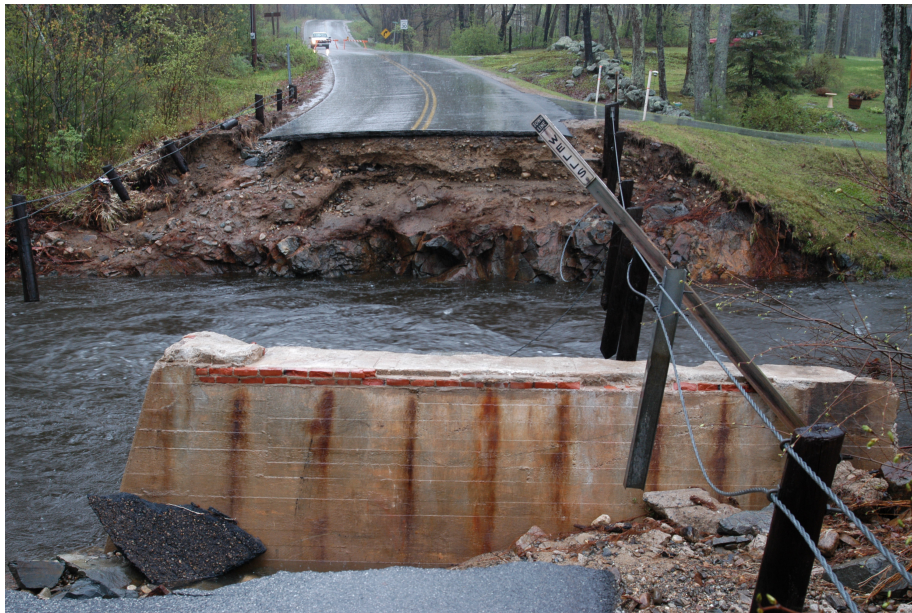
Captain Thomas Road Bridge
