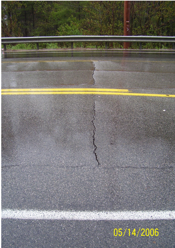
Houston's Curve Bridge (Route One)
