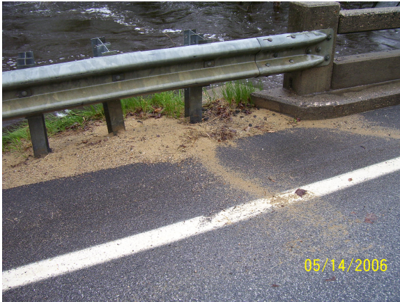
Branch Road Bridge
