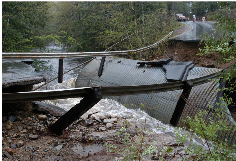
Coles Hill Road Bridge
