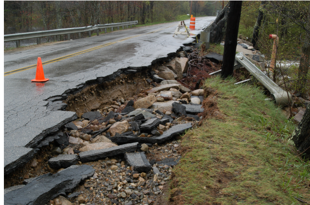
Bragdon Road Bridge
