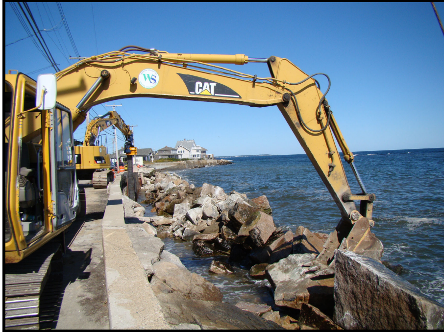
Repair work on Webhannet Seawall
