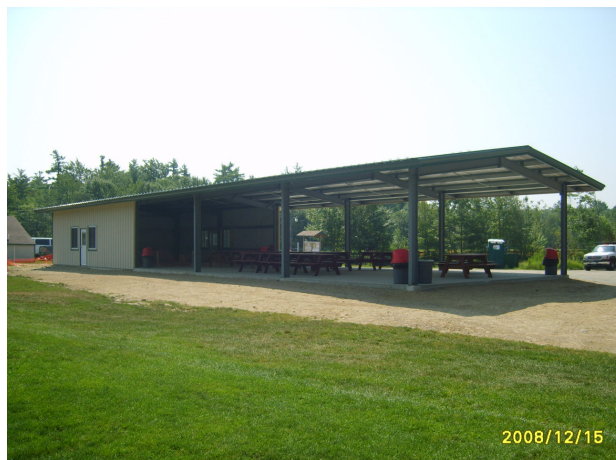
New Pavilion at Wells Parks & Recreation
