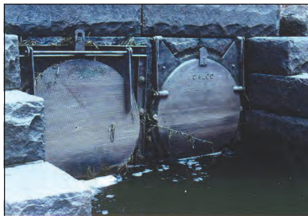
Tide gates deprive many acres of former salt marsh from tidal flow. Photo Michele Dionne.
