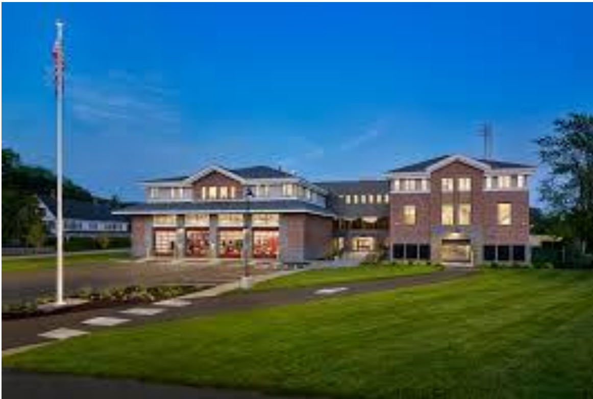
Figure 1 Wells Public Safety Building
